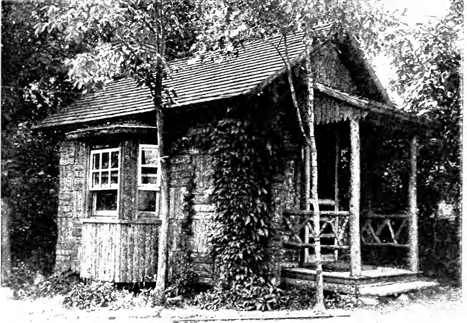
A simple bark cabin in the woods. An unusual effect is obtained by the use of short slabs of bark, arranged vertically and horizontally in squares.
